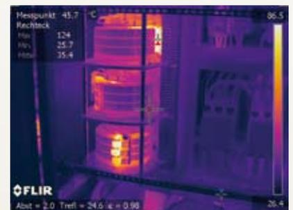
640 x 480 pixel resolution provides sharp imagery of data centers and electrical installations
